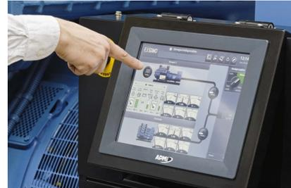
The new APM802 command/control system is specifically designed for operating and monitoring power plants for markets including hospitals, data centres, banks, the oil and gas sector, industries, IPP, rental and mining. This unit is available as standard on all generating sets from 275 Kva designed for coupling. It is optional on the rest of our range.
